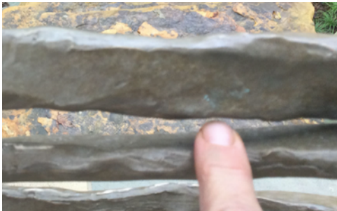
Detail of green corrosion on gate.
