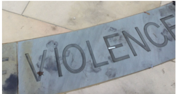
Detail of staining on stone and of debris collecting in engraving..
